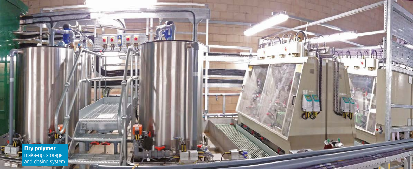
AeroWet 100 + 0.3m³ INT* polymer system
